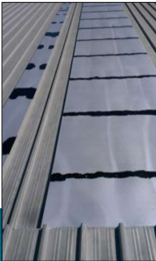
1. RTT Sealant applied to joints and corners
