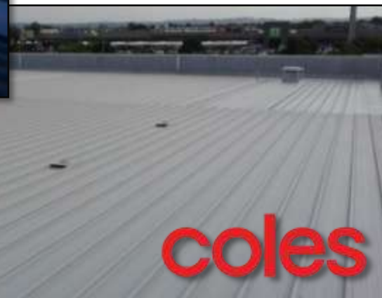
RTT Sealant + Top coat applied to roof to prevent corrosion
