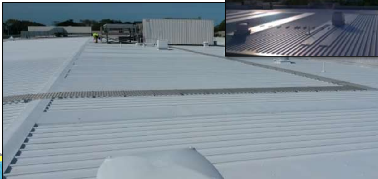
3. Solar Top Coat applied to RTT Sealant
