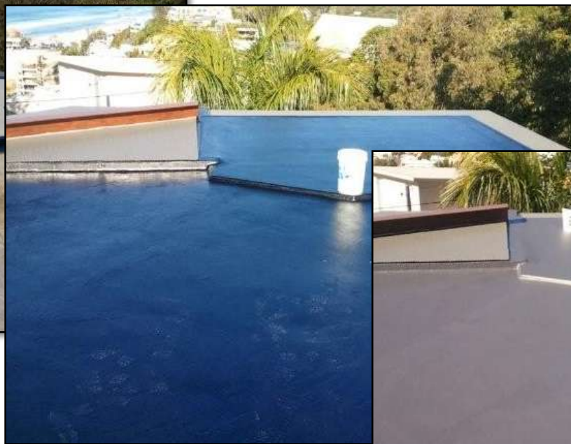
2. RTT Sealant applied to entire area
