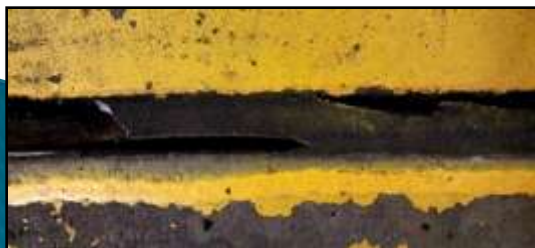
1. Existing seal to be removed
