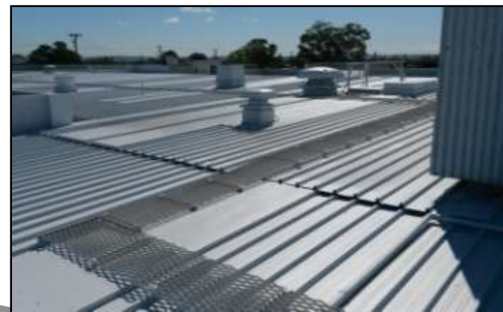
RTT Sealant + Top Coat spray applied
