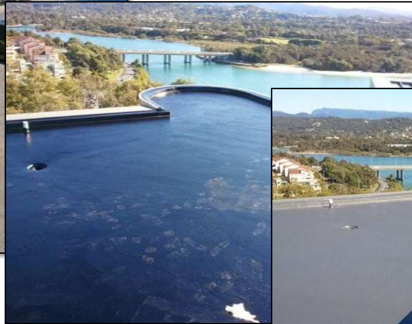
2. RTT Sealant applied to entire area
