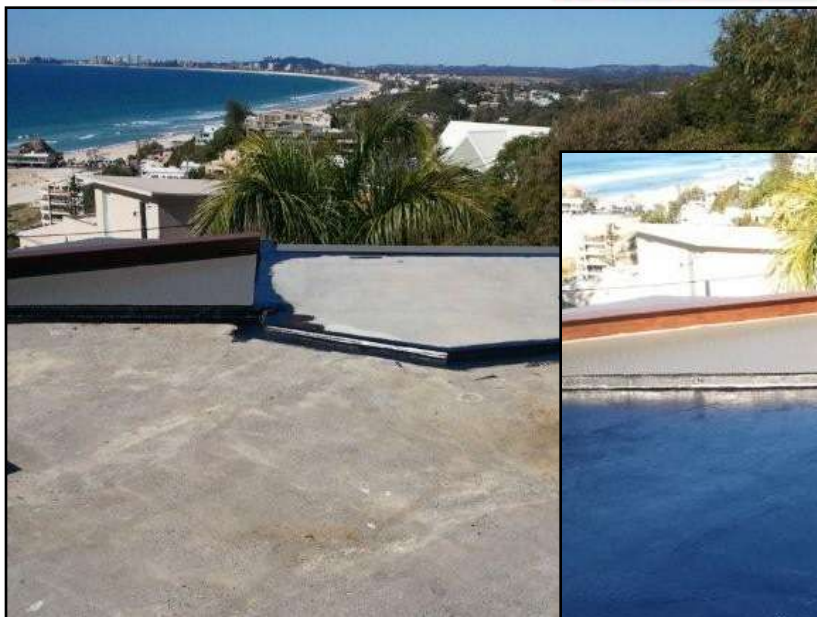
1. RTT Sealant applied to joins and corners
