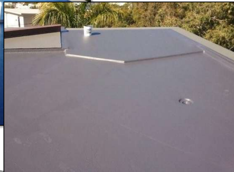
3. Coloured top coat applied to RTT Sealant
