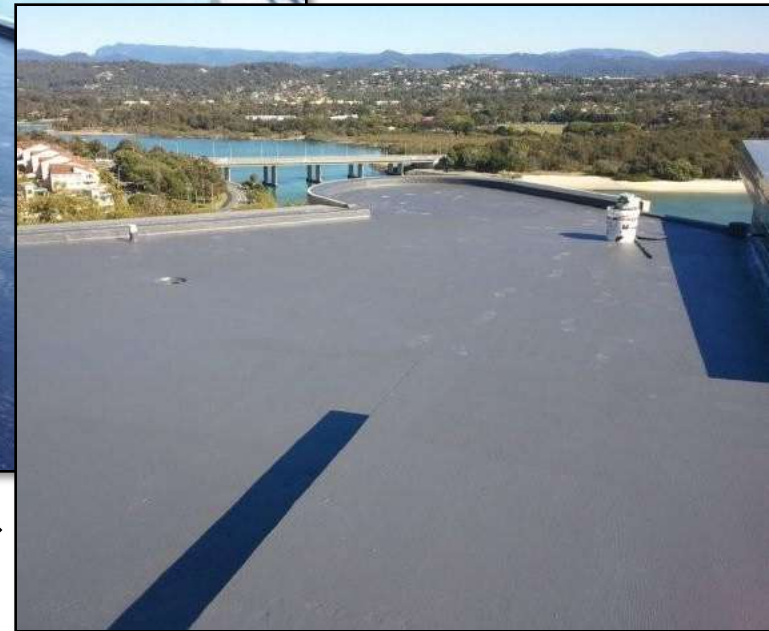
3. Coloured top coat applied to RTT Sealant
