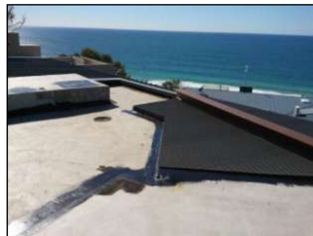
RTT Sealant brush/roller applied
