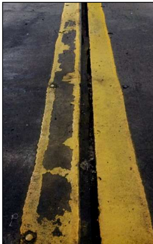
Existing joint sealant to be removed
